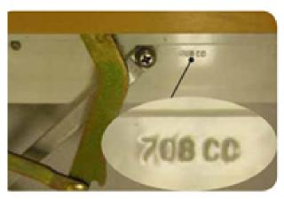
**Unit ID Label**. Windows manufactured between 1998 - 2009 have a Unit ID Label that can be found on interior lower corner of the glass of each window, and looks like this:
